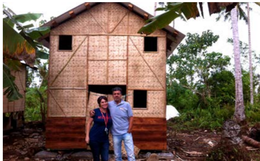
Heidi Cockram and Alberto Livoni in front of partially completed house after Typhoon Haiyan
